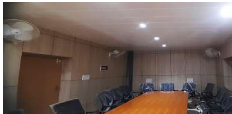
Figure 6. LED enabled well-equipped conference hall at Bangabasi Evening College
